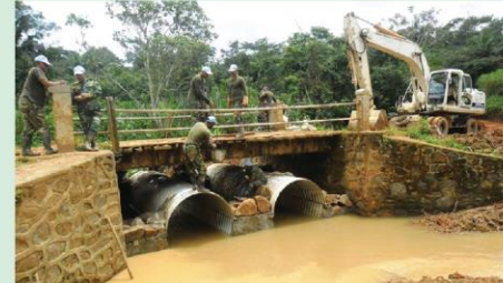
Bangladesh Army Engineer Contingent is Constructing Culvert in DR Congo
